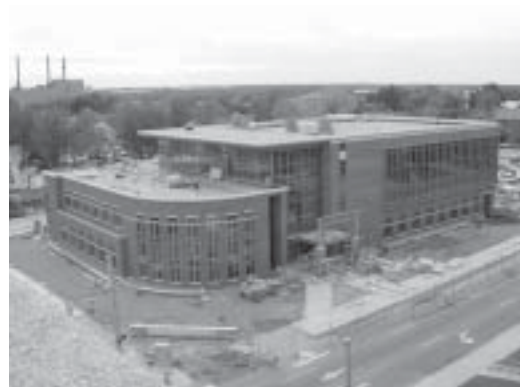
Construction in progress
